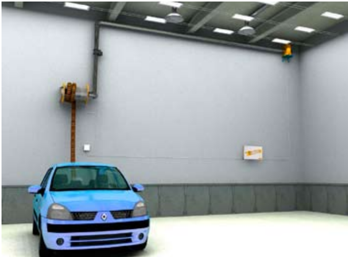
Hose reels with micro-switches MSR-24/2, fan starter SA-24 and TEV fan.
