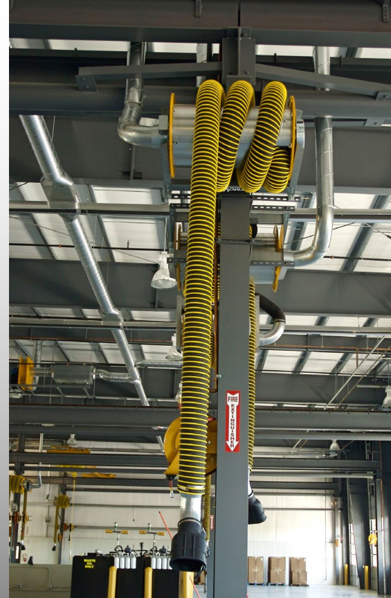
Pictured to the right: EF2 Exhaust Hose on an a Spring-Operated Exhaust Reel (SER) Hose Reel
