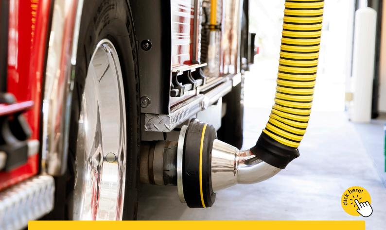
The Magnetic Grabber<sup>®</sup> is a patented vehicle exhaust removal device and winner of the reddot design award.
